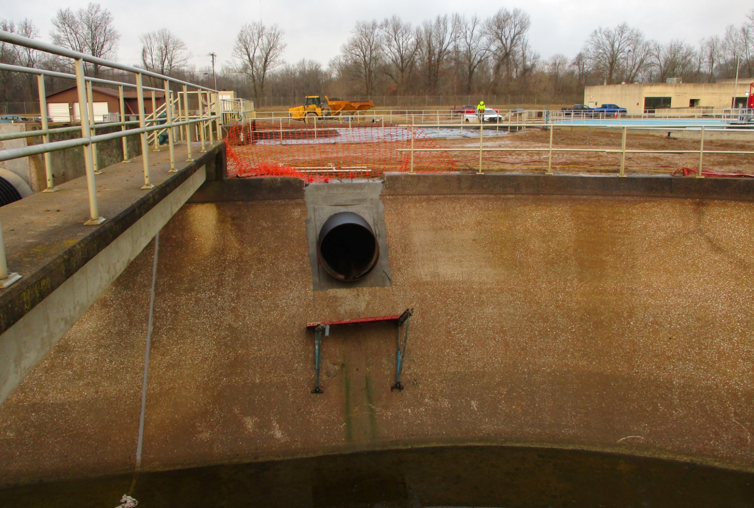
Oxidation Ditch No. 2- Photo 3
