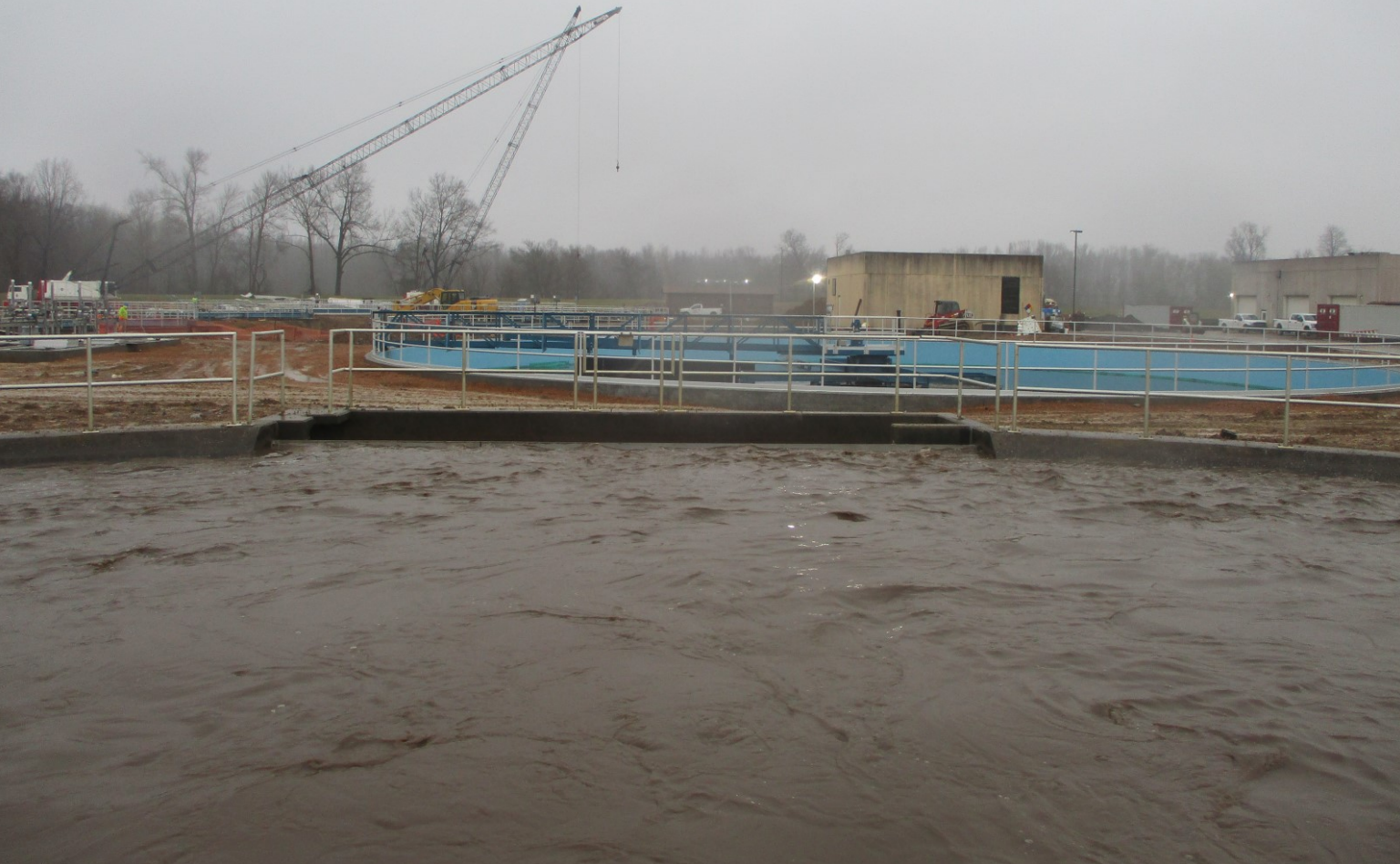
Oxidation Ditch No. 2 - Photo 4
