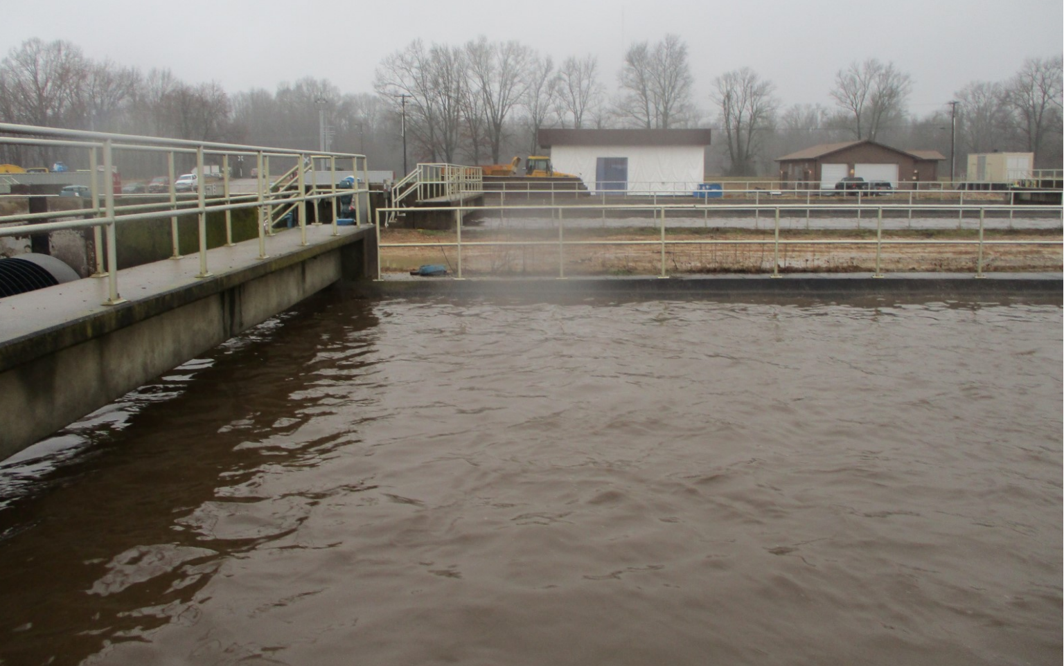
Oxidation Ditch No. 2 - Photo 2
