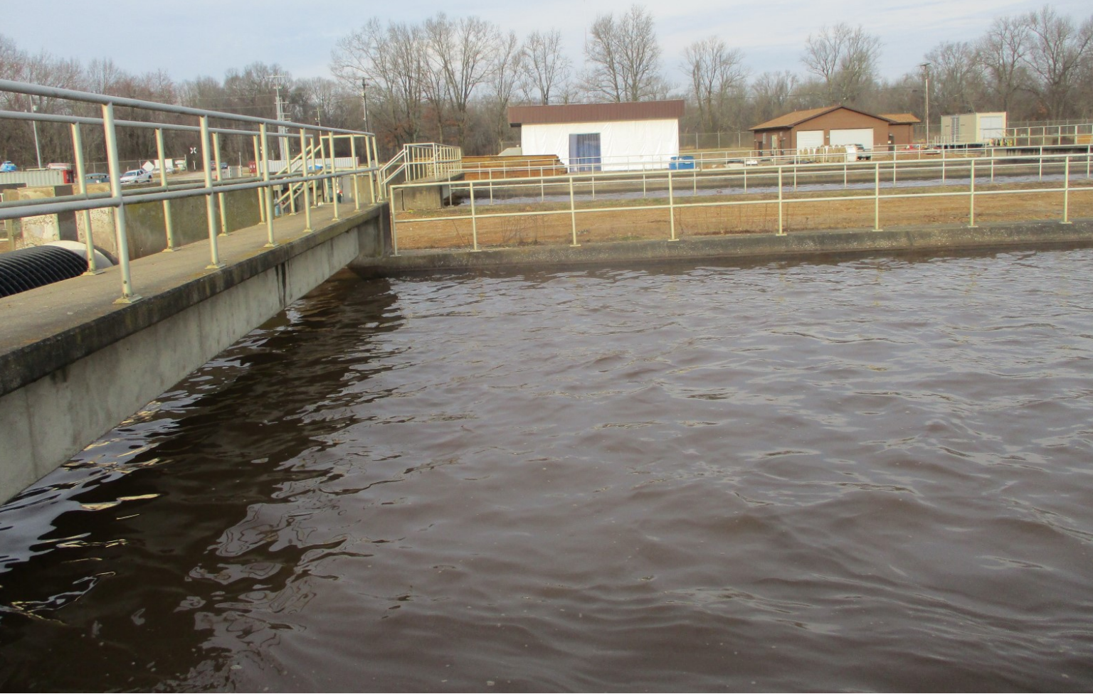
Oxidation Ditch No. 2 - Photo 2
