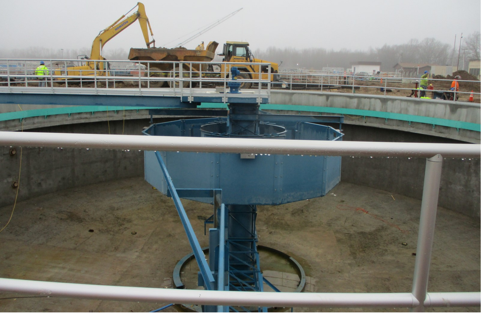
Clarifier No. 6 - Photo 2
