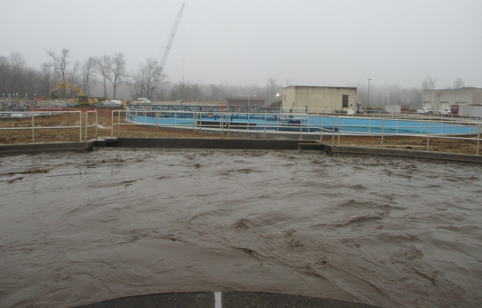
Oxidation Ditch No. 2 - Photo 4
