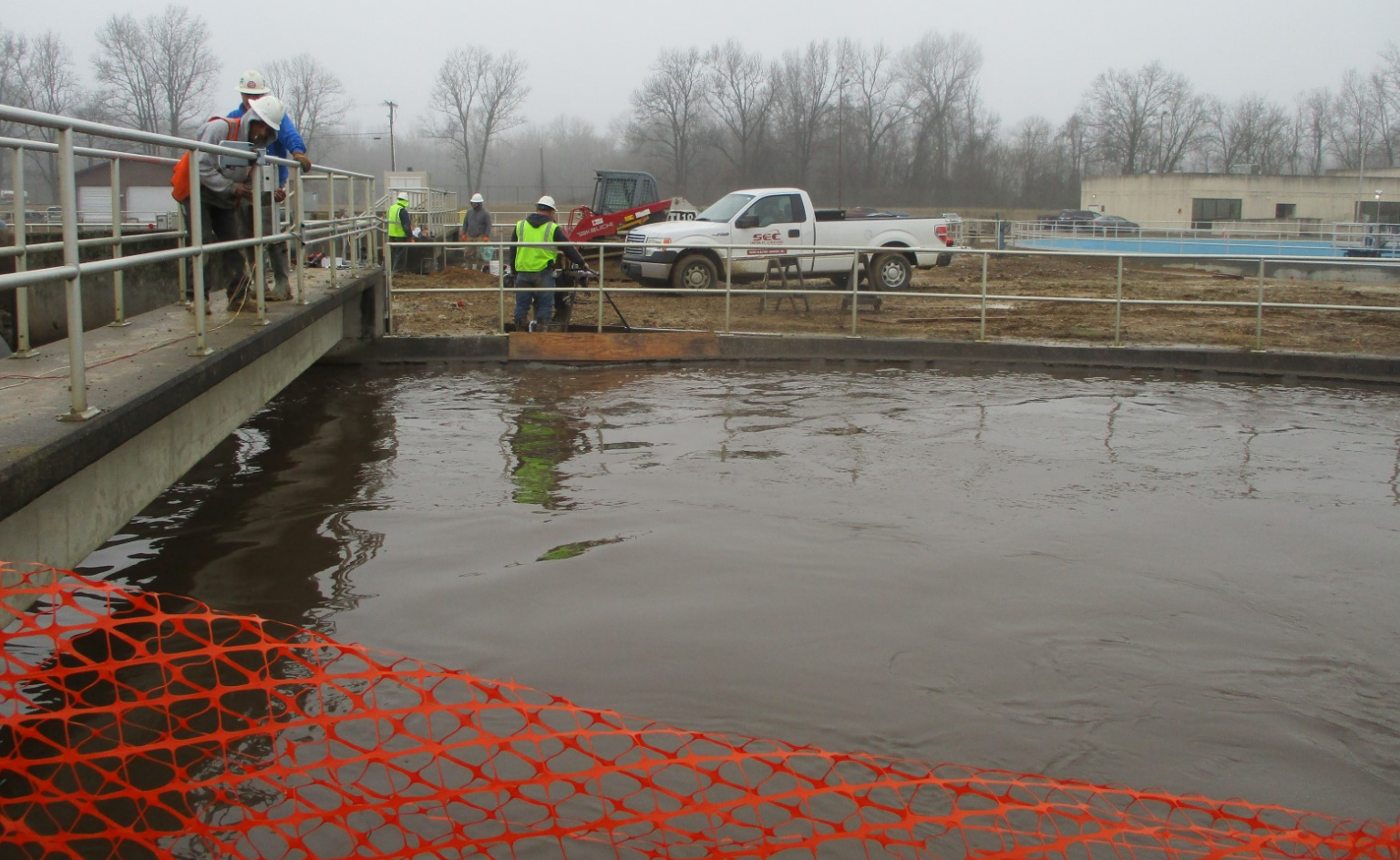
Oxidation Ditch No. 2 - Photo 3
