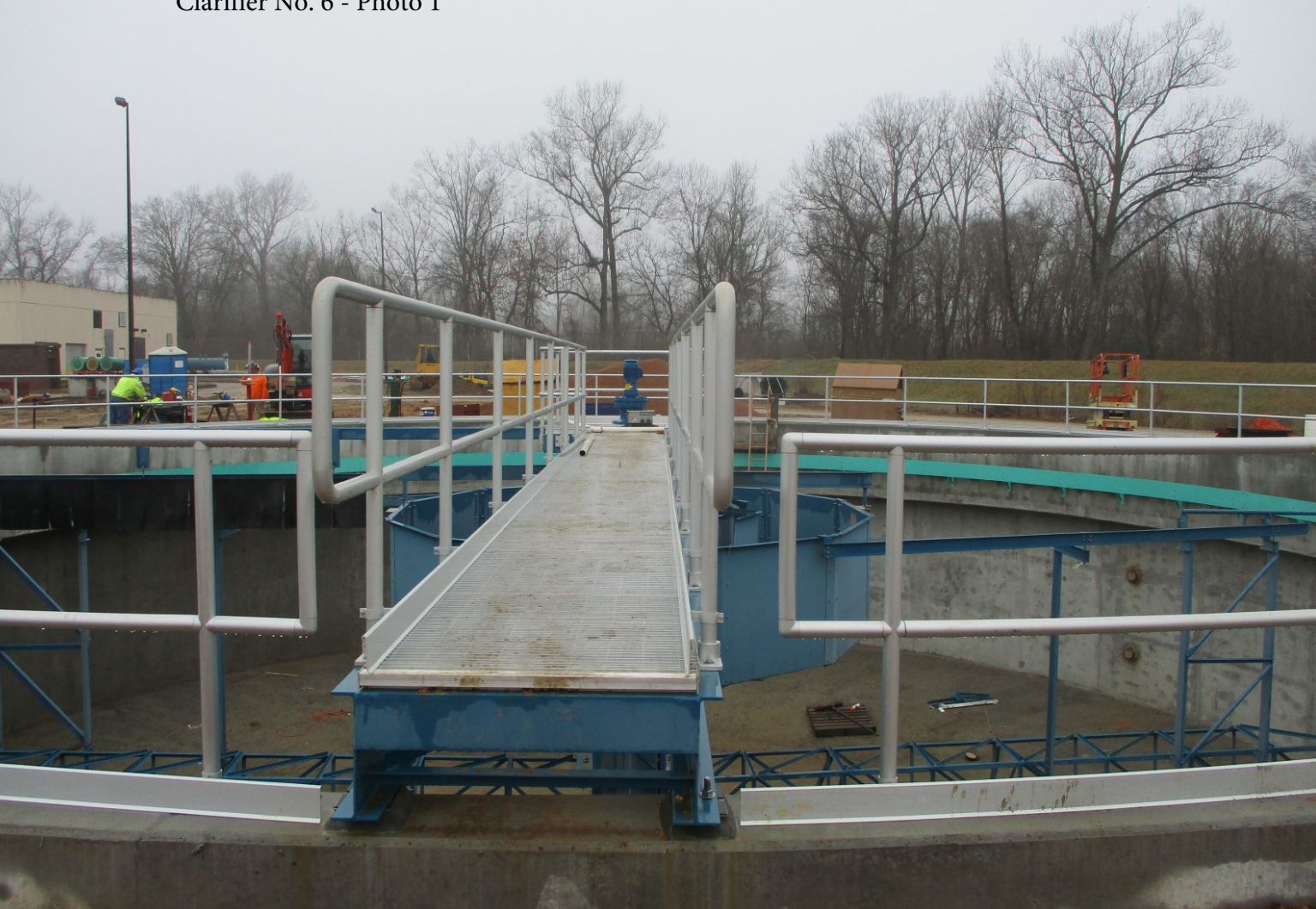
Clarifier No. 6 - Photo 1
