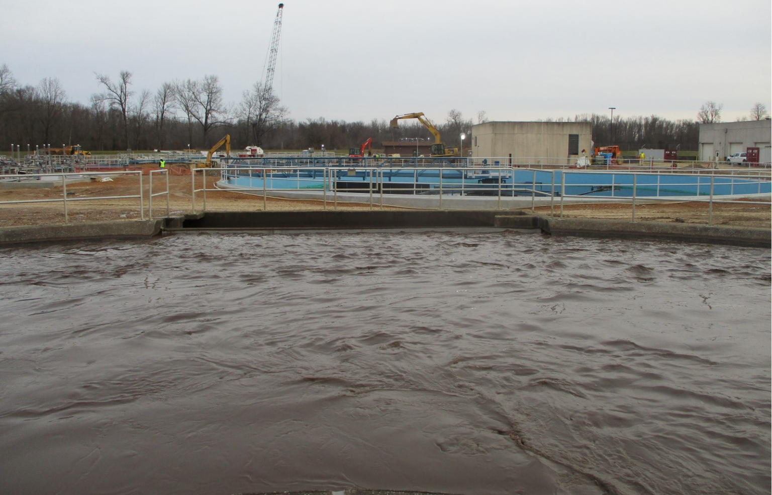
Oxidation Ditch No. 2 - Photo 4
