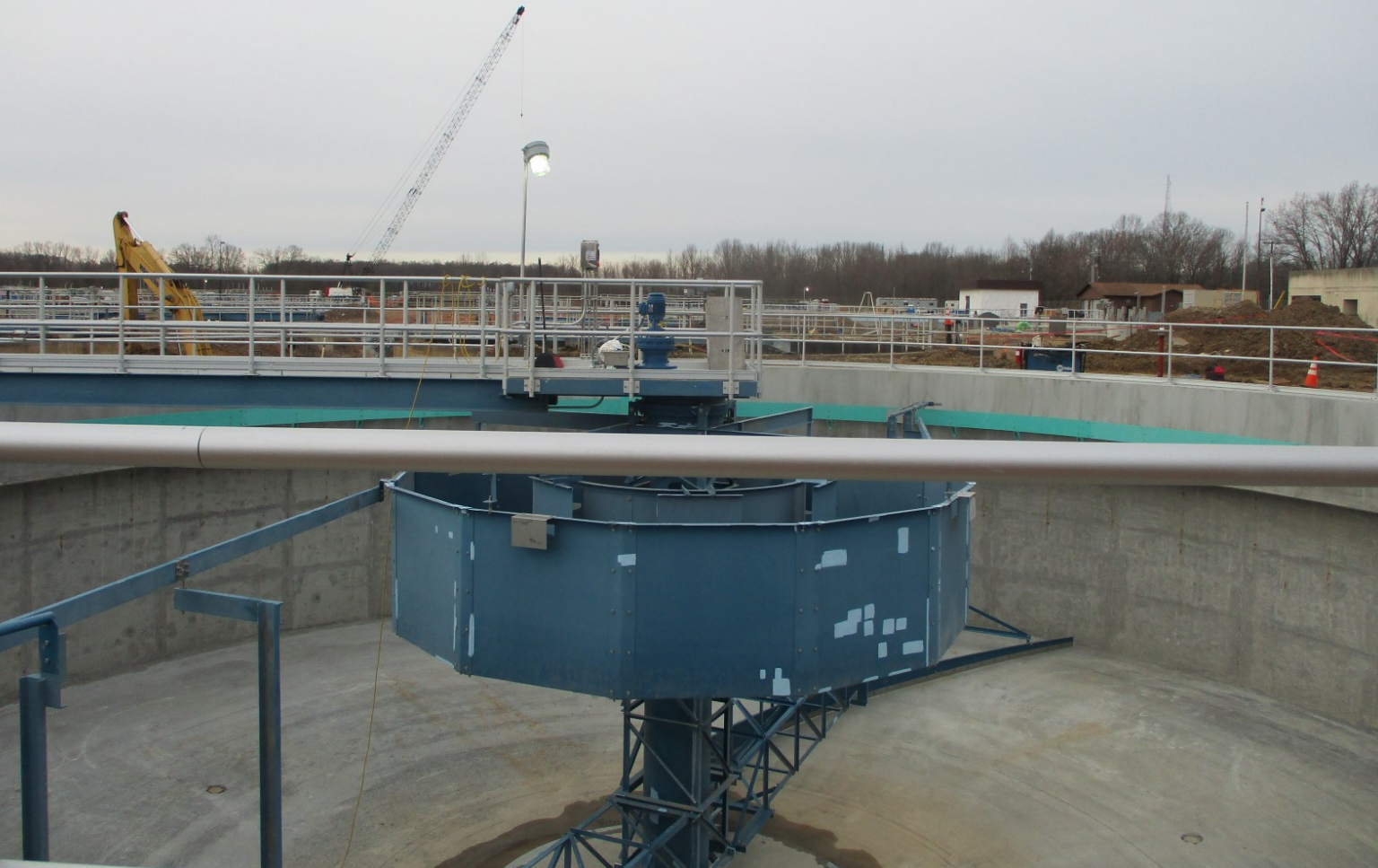
Clarifier No. 6 - Photo 2
