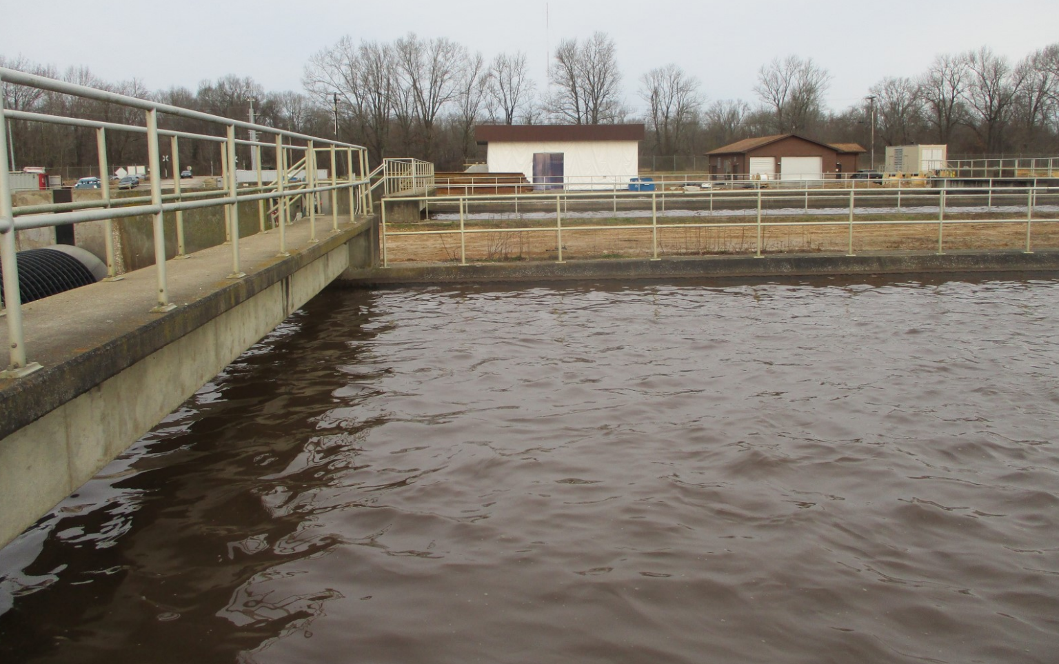
Oxidation Ditch No. 2 - Photo 2
