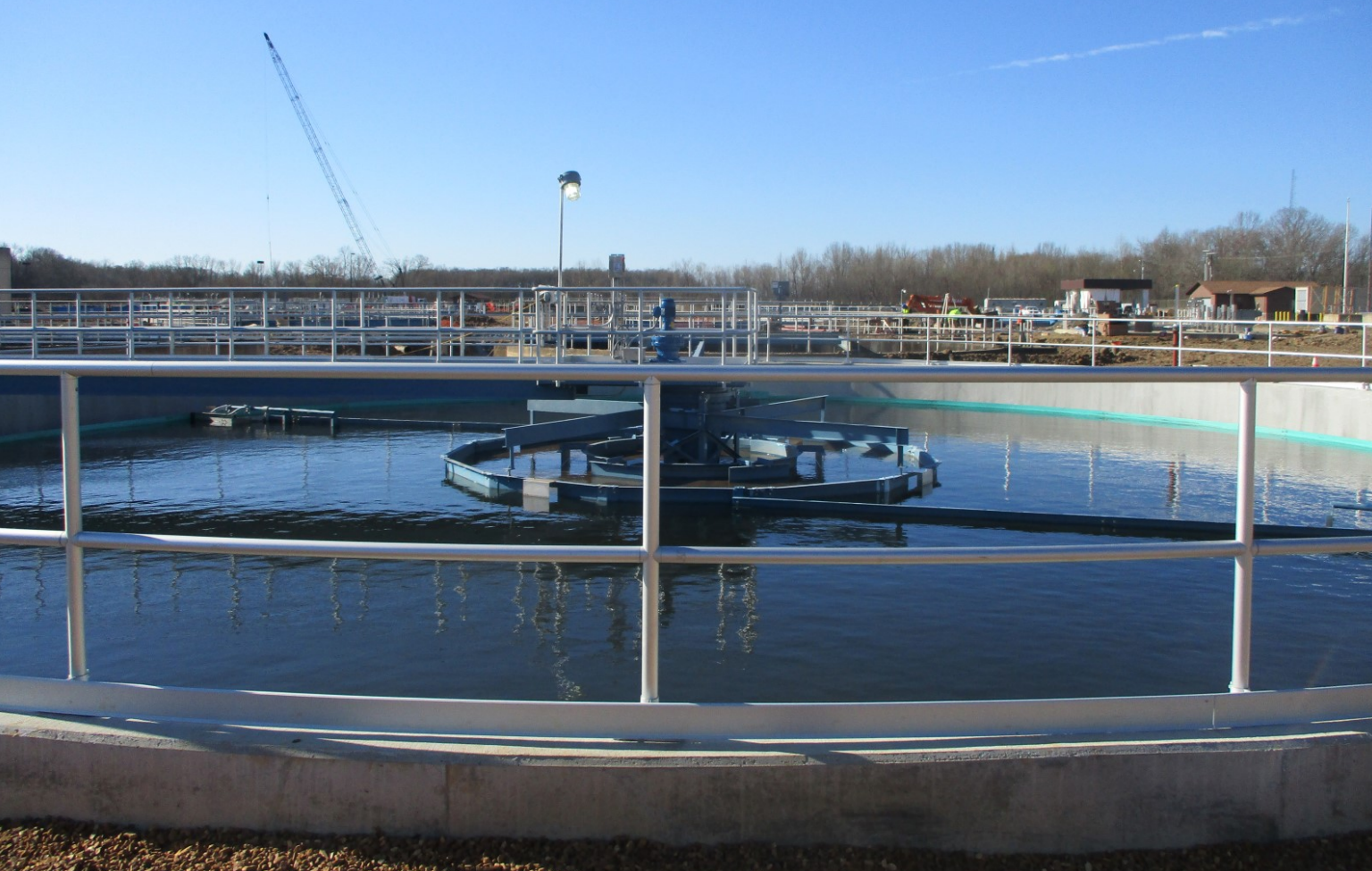
Clarifier No. 6 - Photo 2
