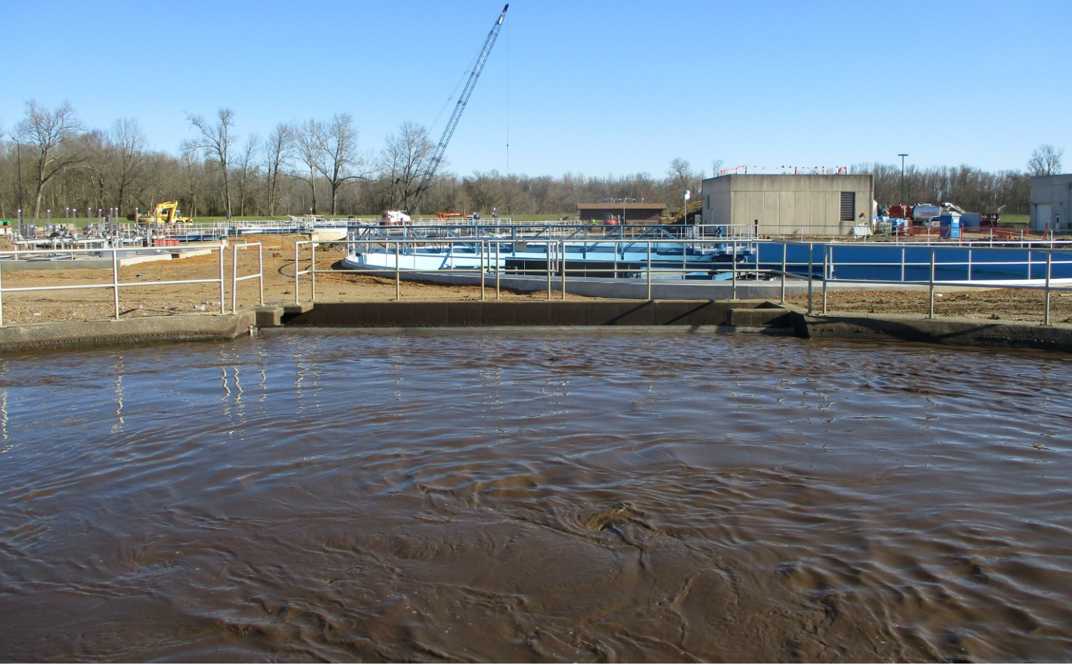
Oxidation Ditch No. 2 - Photo 4
