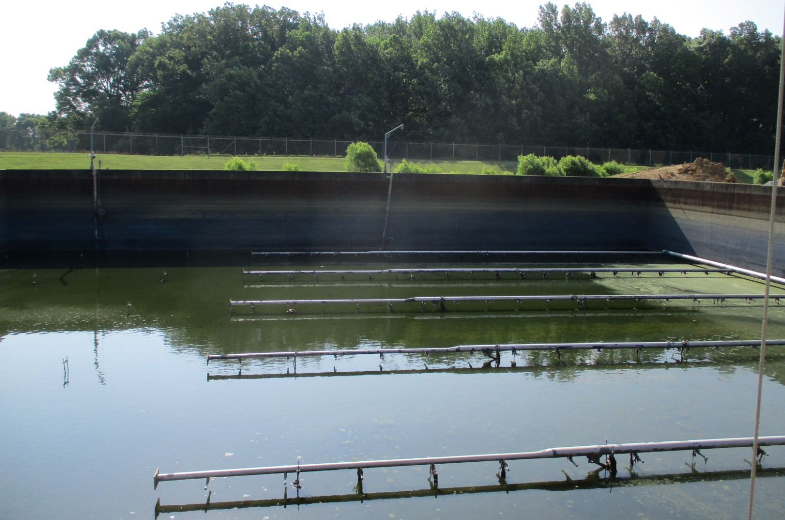
Interchange Tank - Photo 1
