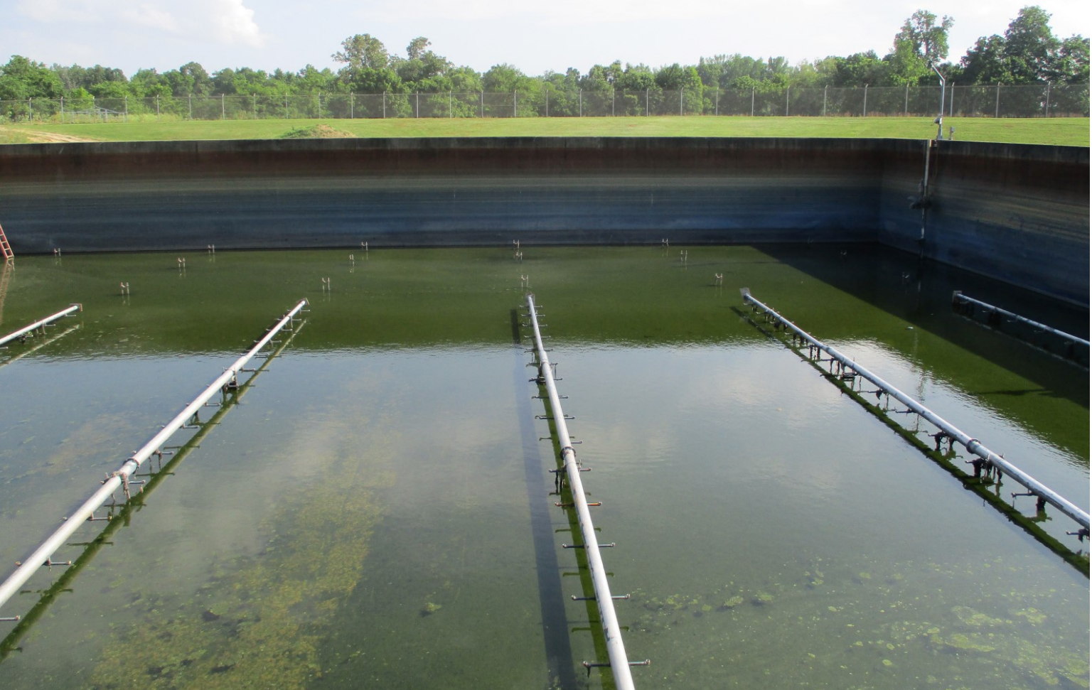
Interchange Tank - Photo 2
