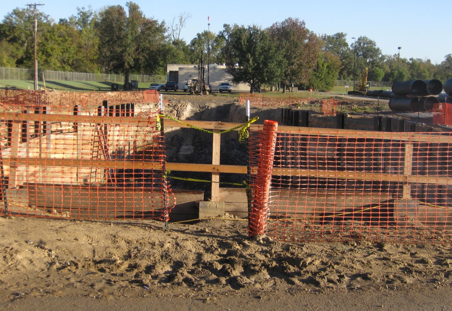
Pretreatment Structure Excavation - Photo 2
