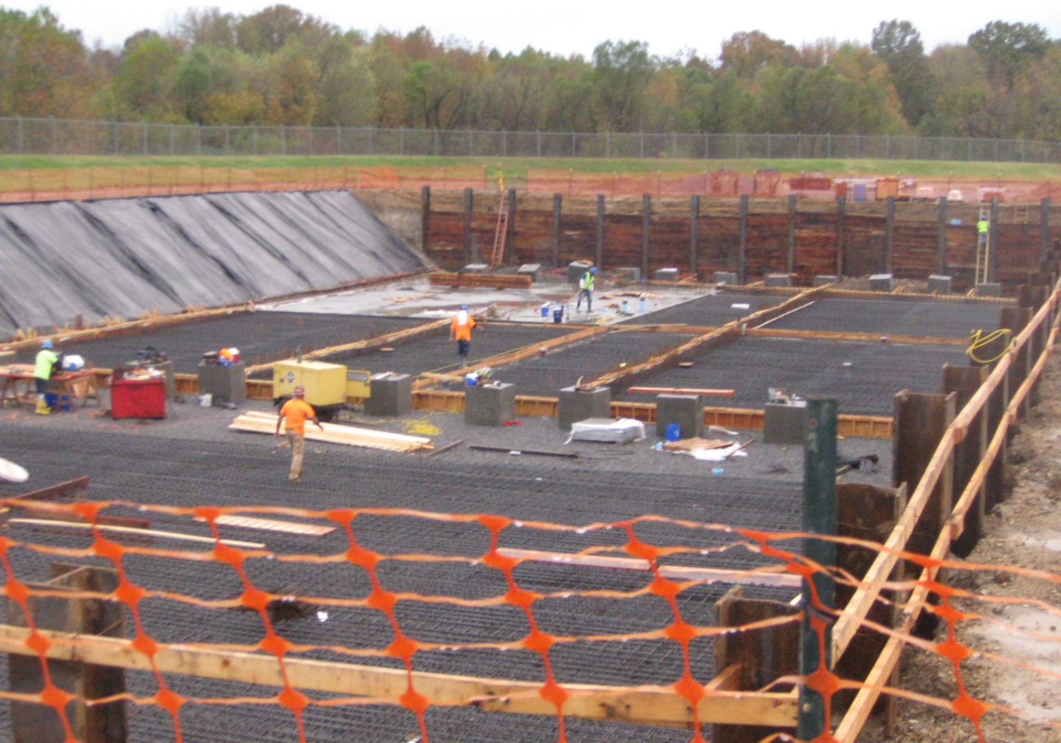
Vertical Loop Reactor - Photo 4
