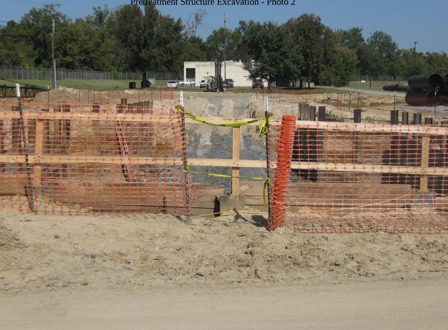
Pretreatment Structure Excavation - Photo 2
