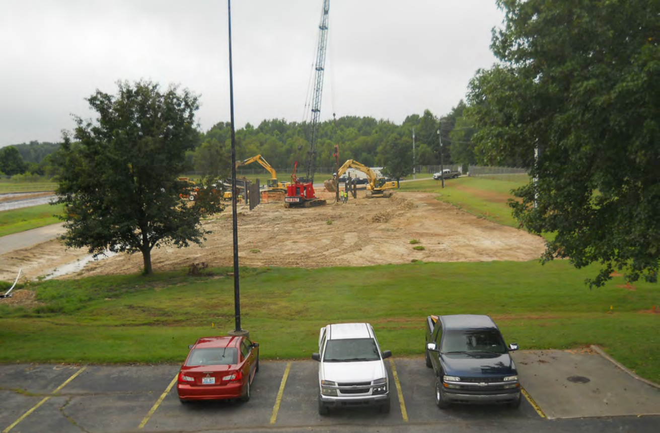
Pretreatment Structure Excavation - Photo 8
