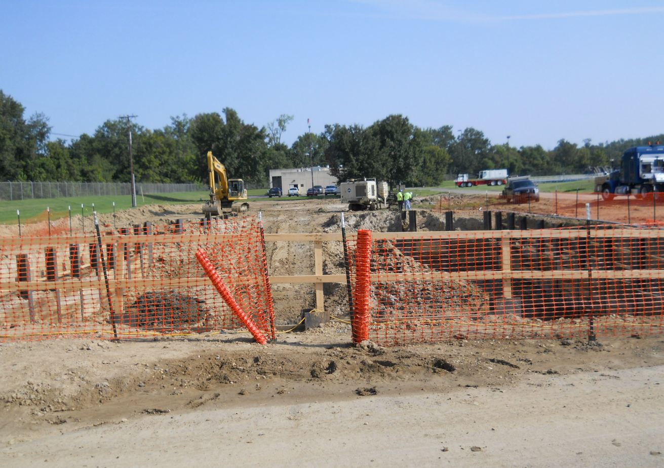
Pretreatment Structure Excavation - Photo 1
