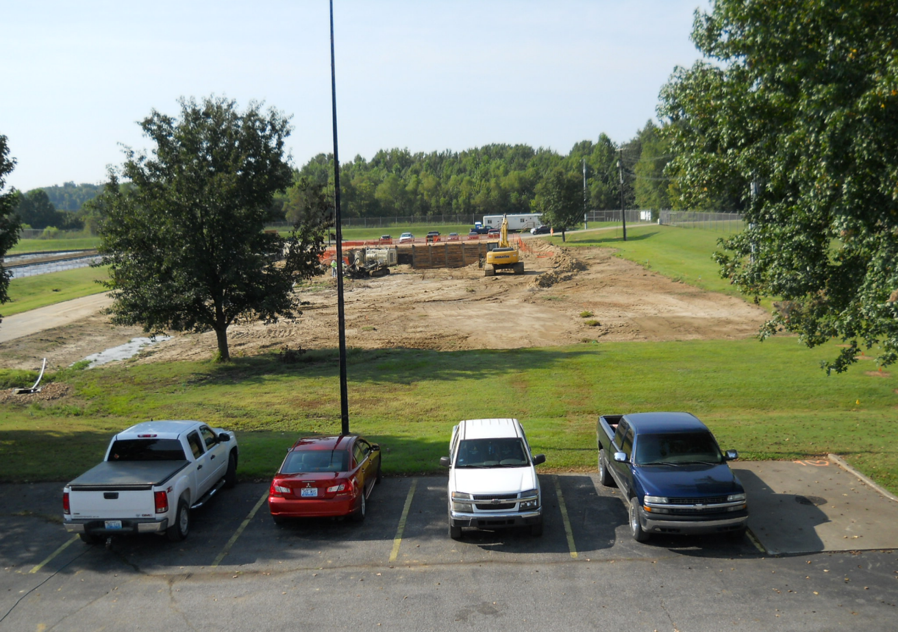
Pretreatment Structure Excavation - Photo 3
