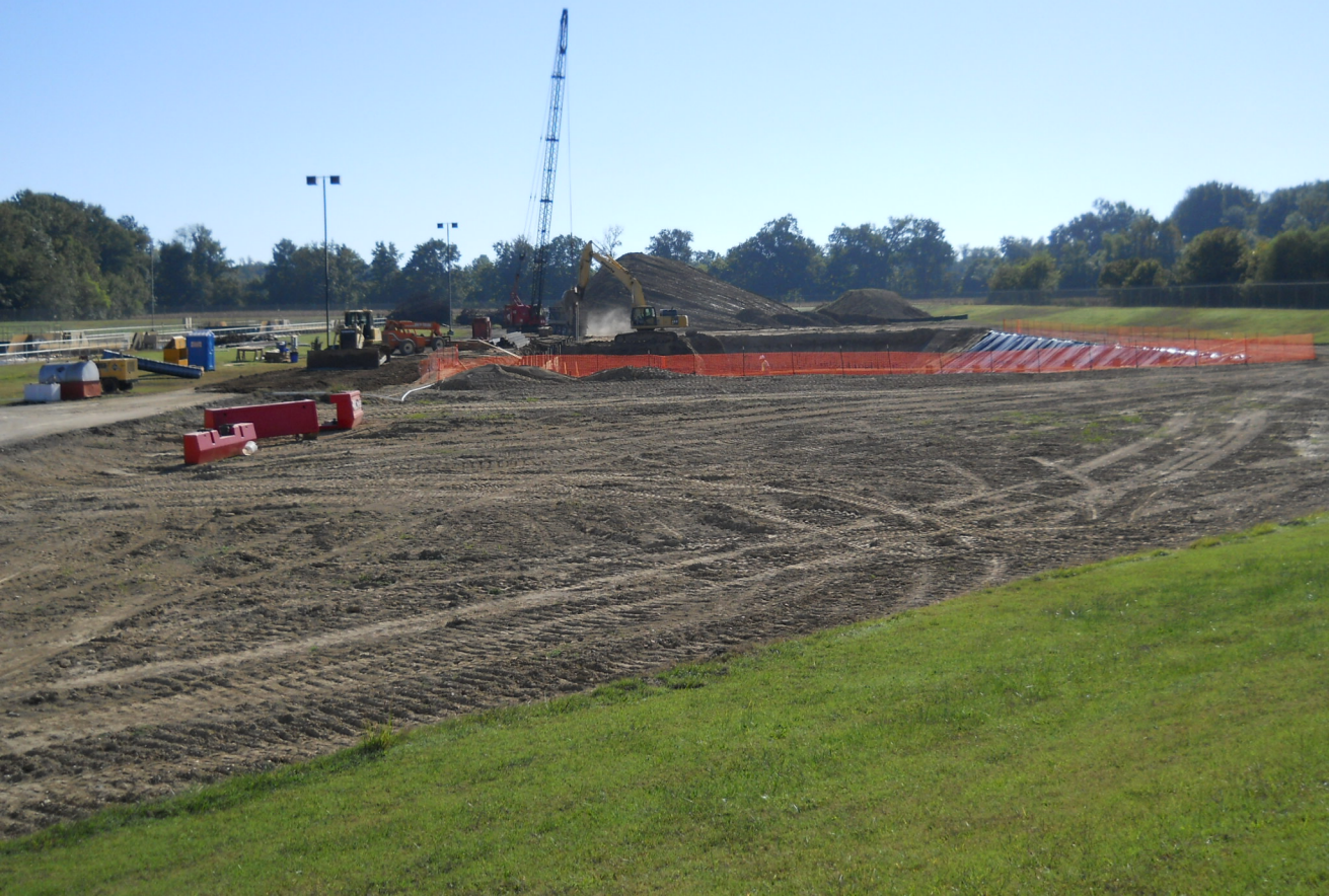
Vertical Loop Reactor Excavation - Photo 4
