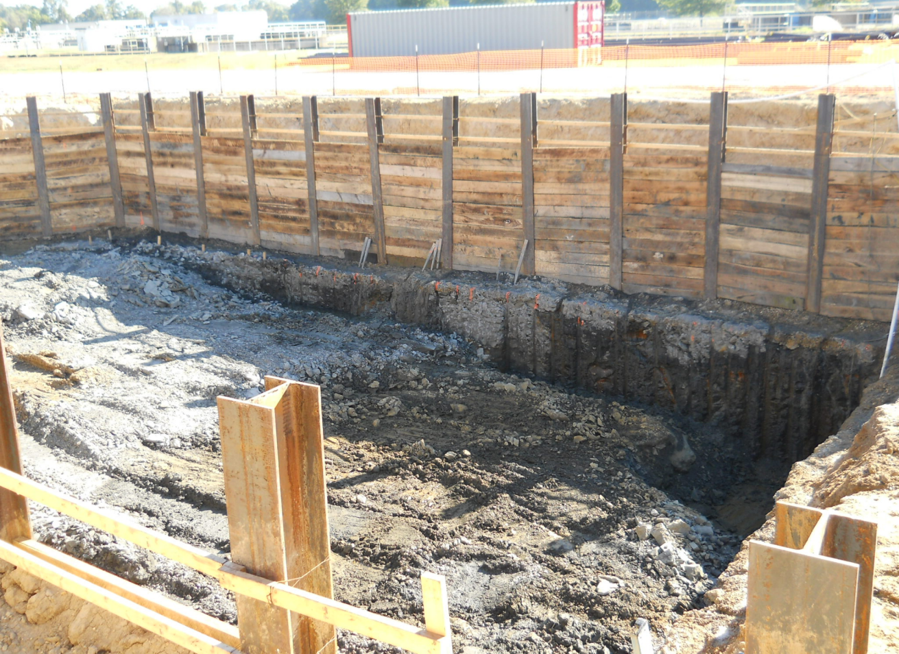
Pretreatment Structure Excavation - Photo 2
