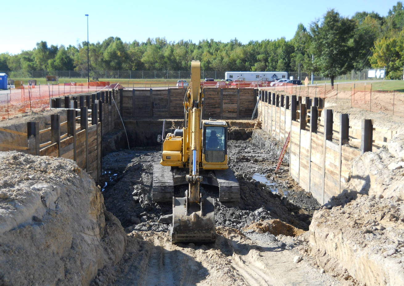
Pretreatment Structure Excavation - Photo 1
