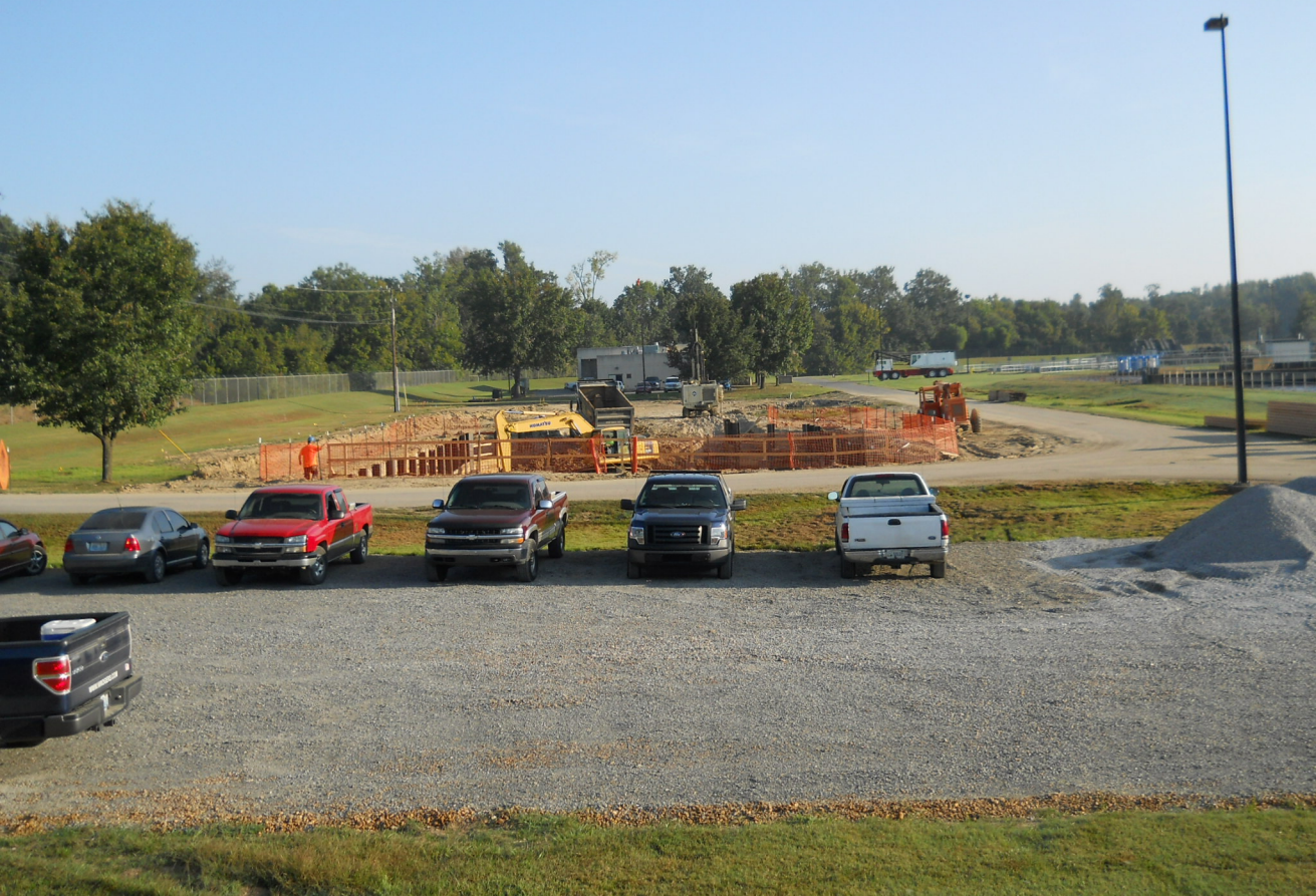
Pretreatment Structure Excavation - Photo 1
