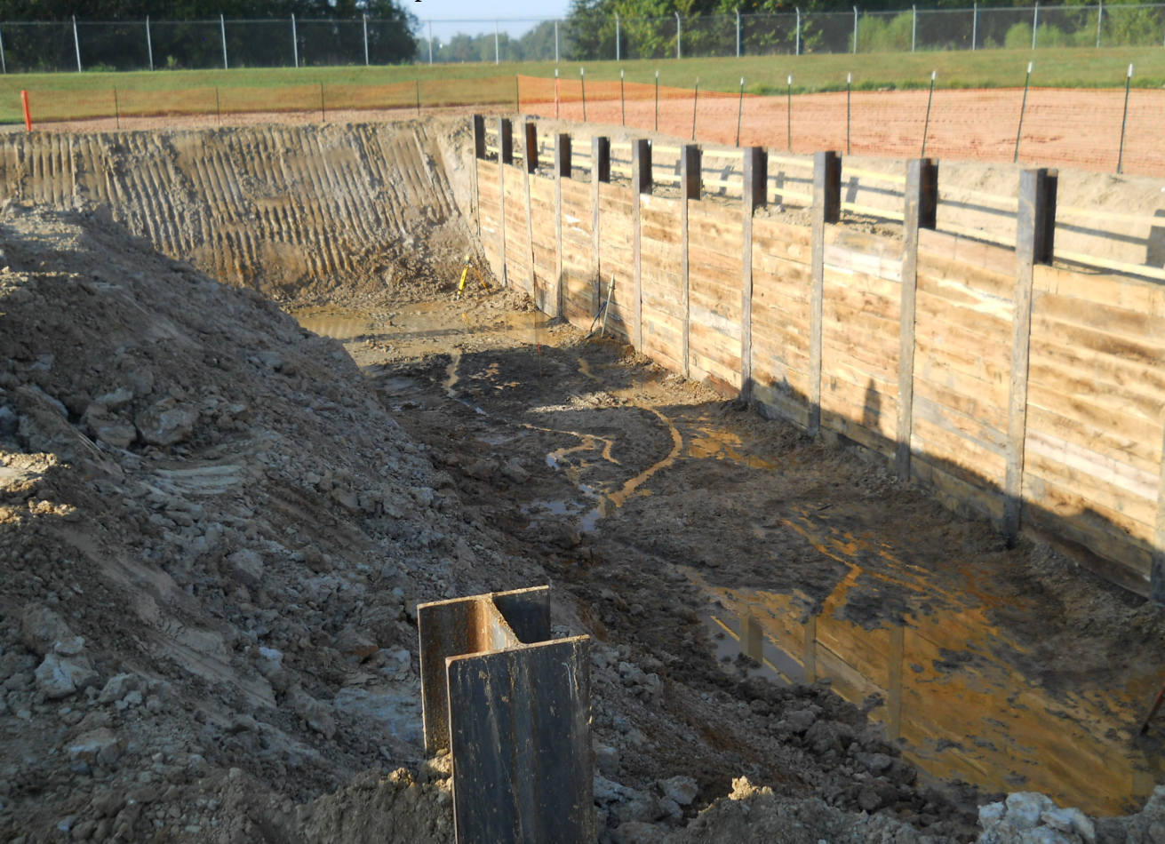
Vertical Loop Reactor Excavation - Photo 4
