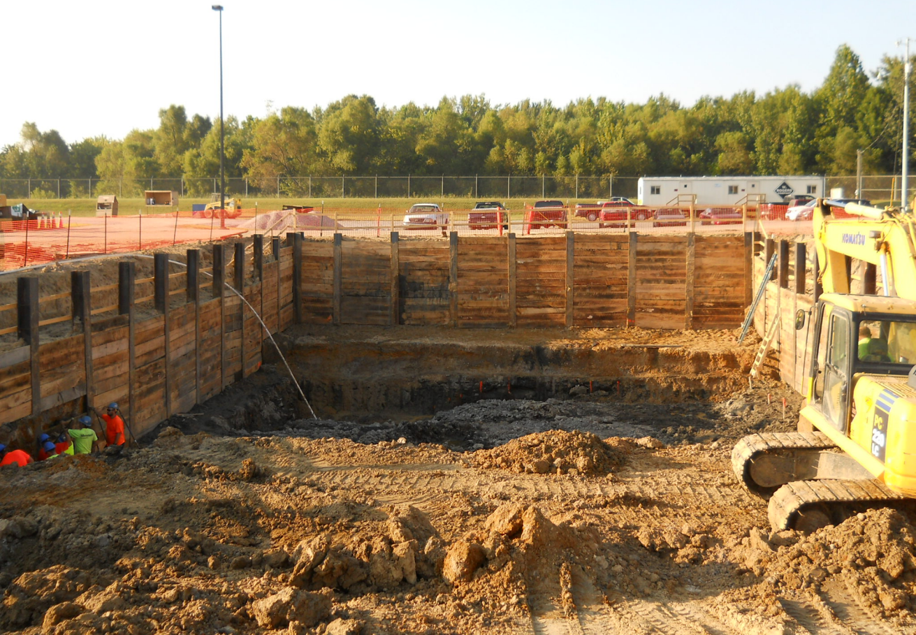
Pretreatment Structure Excavation - Photo 3
