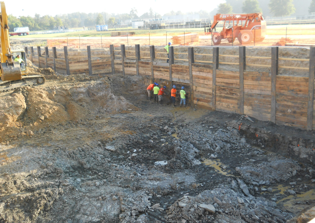
Pretreatment Structure Excavation - Photo 2
