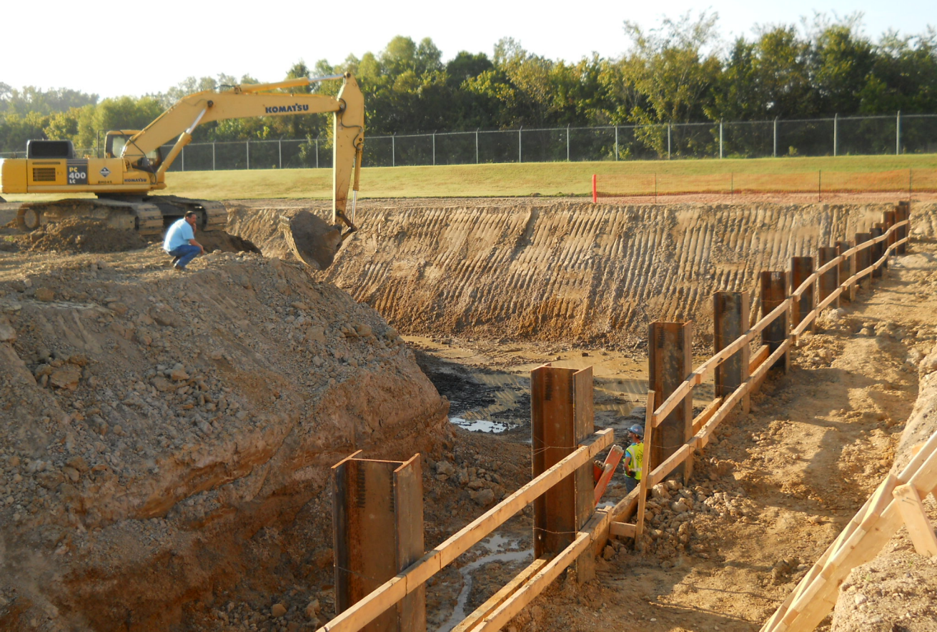
Vertical Loop Reactor Excavation - Photo 2
