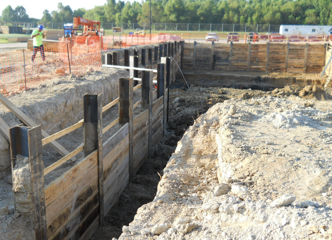
Pretreatment Structure Excavation - Photo 4
